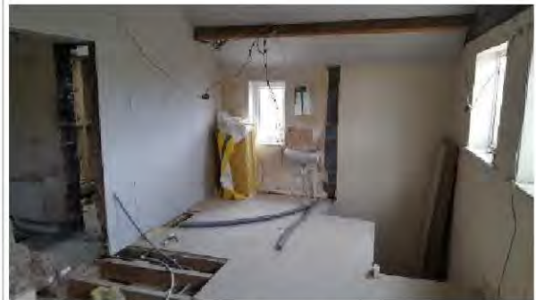
First Floor Rear Storage
