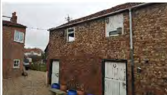
Access to Rear Car Park
